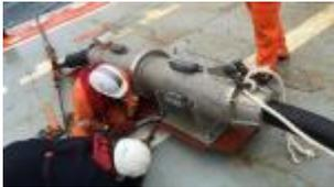
On 21 September 2015, Sabella D10 hydrokinetic turbine was connected to the submarine cable linked to the isle of Ouessant. It will be connected to the network of the island in the coming days, becoming the first tidal turbine connected to an electricity grid in France. The operation consisted to connect the underwater cable from the turbine to the cable submerged in the island. A delicate operation... [Read more](#)
