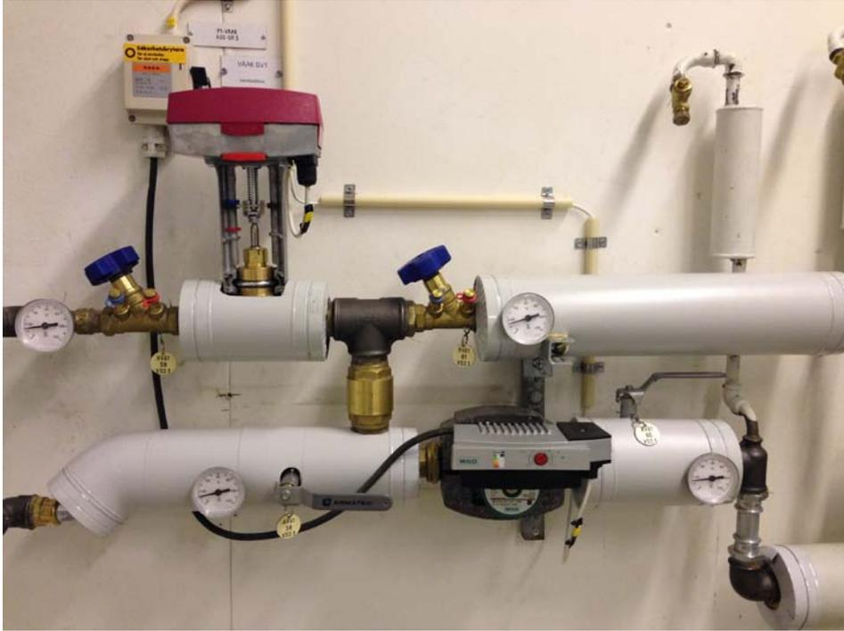
Image 1. New control equipment for heating control to make sure that the right amount of hot water is supplied at every moment.
