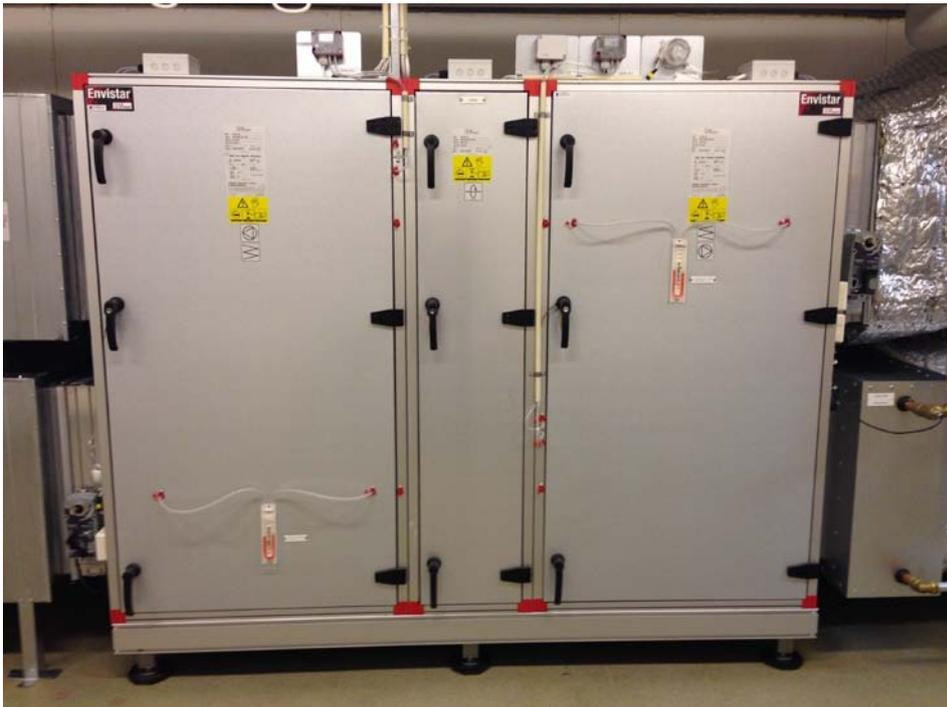
Image 2. New ventilation unit with heat recovery and energy-efficient fans.
